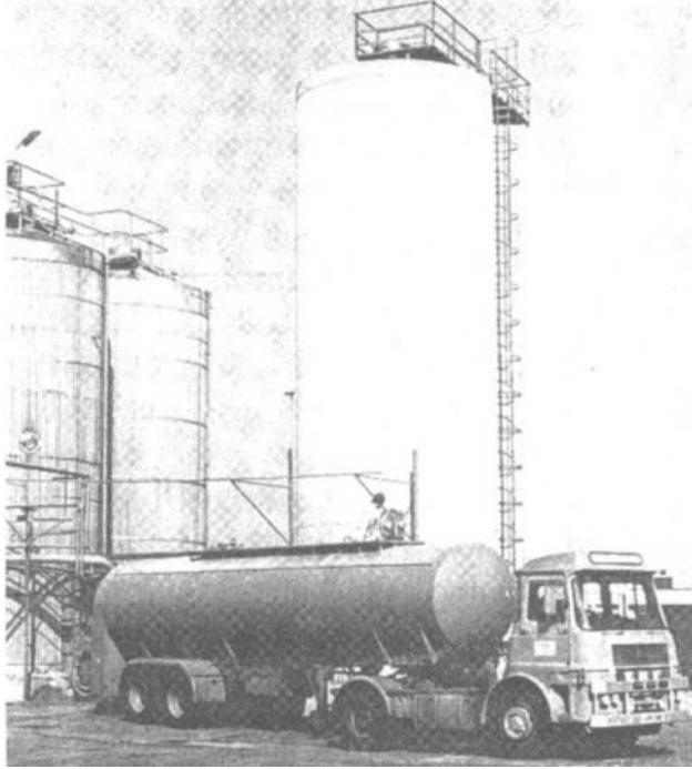
Figure 2.7. These insulated storage silos are used to store raw milk prior to processing. The larger silos hold up to 30,000 gal of milk, whereas the smaller ones hold up to 25,000 gal. (Reproduced by courtesy of the Milk Marketing Board, Davidstow.)
